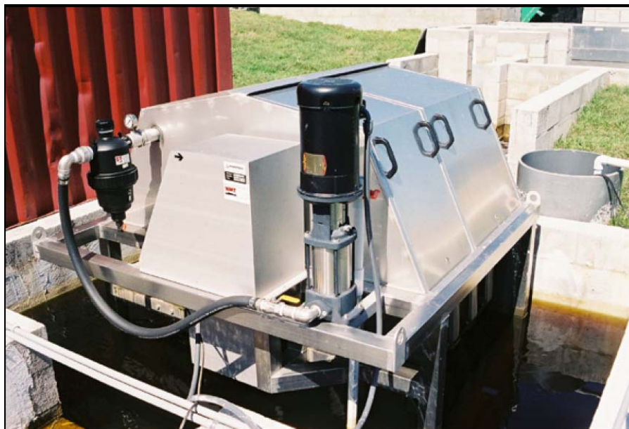
Illustration 1. Hydrotech Model 1704 Discfilter (10 micron) at S-154 Algal Turf Scrubber® system in Okeechobee County, Florida.
